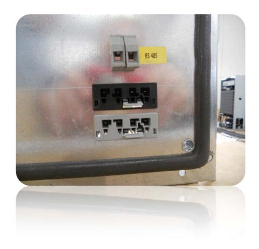
Polyurethane seal applied by continuous molding: by our background on enclosures we derived this sealing system, that reduces mounting operations and give a better fit of our coolers.
